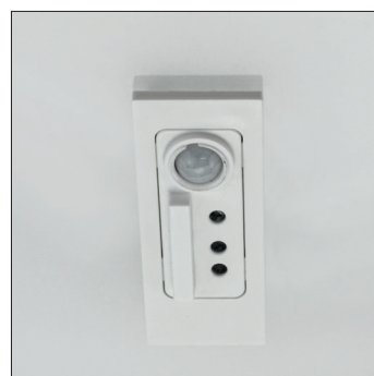
XC daylight&occ sensor
